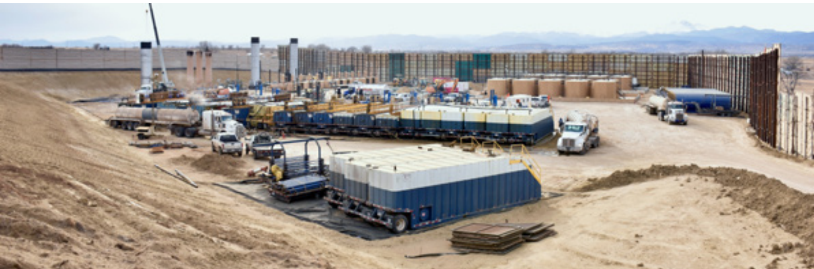
MARKHAM PAD IN THE WATTENBERG FIELD, USA
