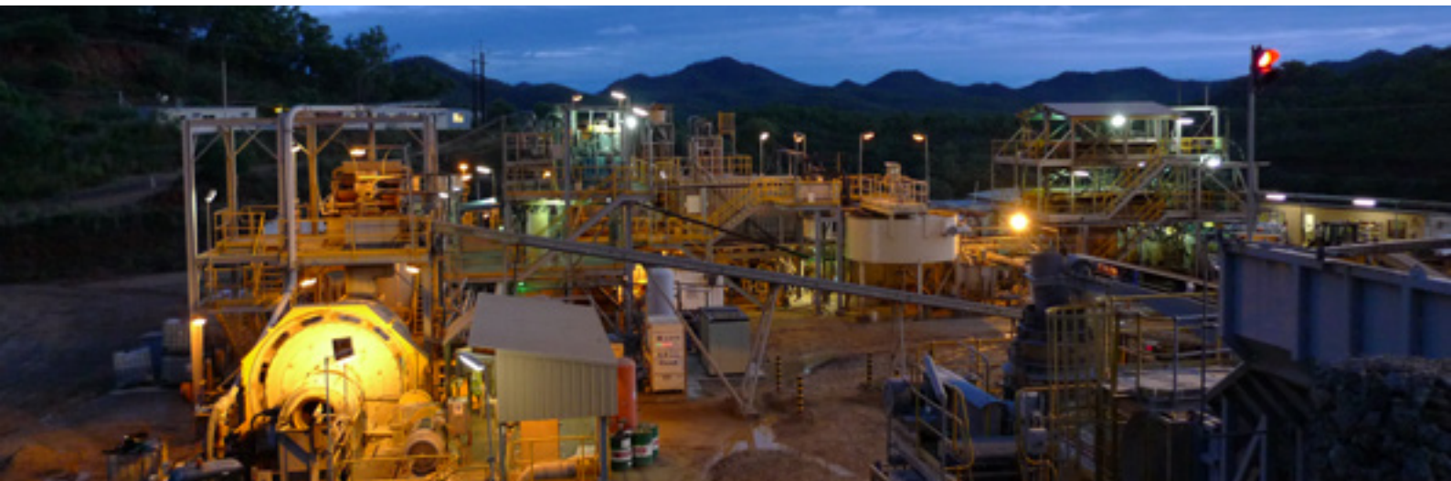
PROCESSING PLANT AT WOLFRAM CAMP MINE, AUSTRALIA
